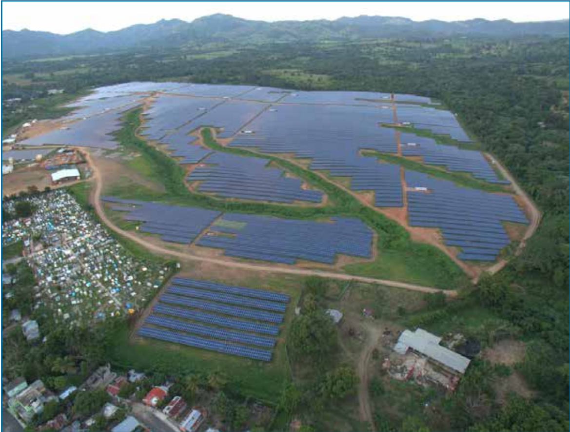
Monte Plata Solar farm. Capacity 30 mW
